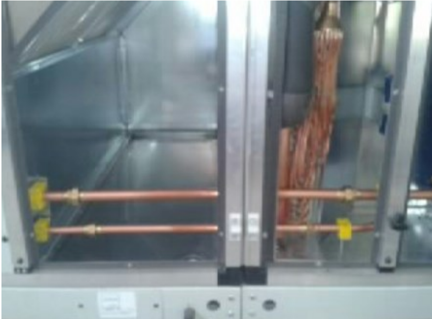
Connector connection was done of suction and discharge lines for with plate type recovery unit
